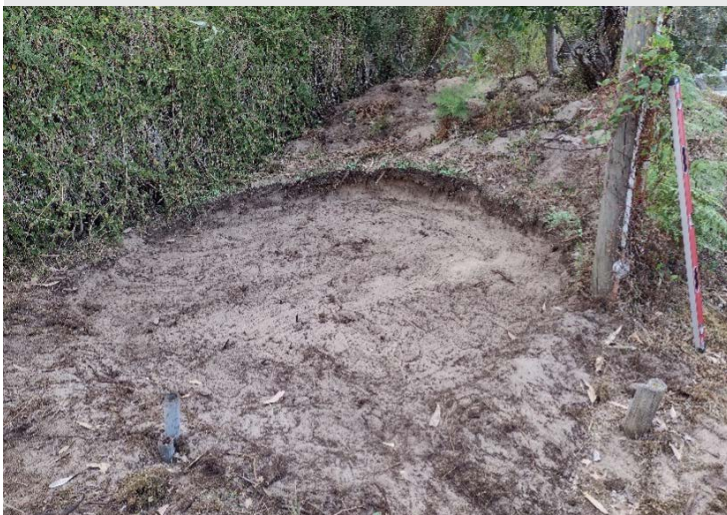
Getting ready for the new 10,000l water tank.
